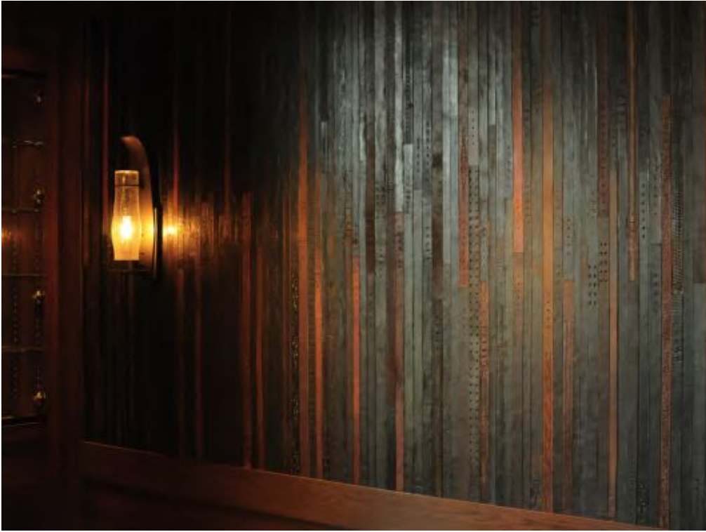
Vintage leather belt walls made for a restaurant in Orange County, California. The flooring and wall panelling are a bespoke product designed for use in private and commercial spaces.
